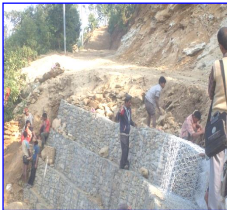
Gabion wall works at Tandarn VDC, Gorkha
